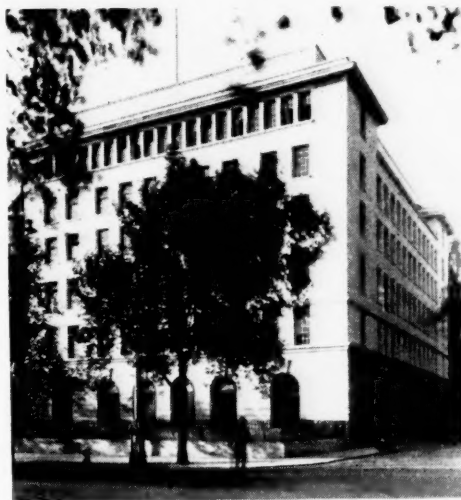
The radiant heated Daily Mail building, one of eight London newspapers radiant heated with panels. The ninth is electrically radiant heated.
