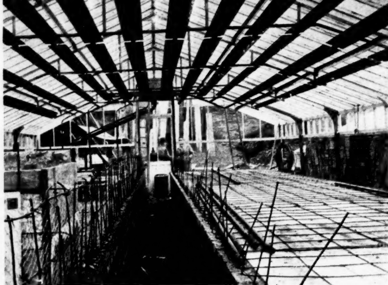
A French greenhouse radiant heated. Note the reflectors over the pipes from which the radiant heat is derived.
