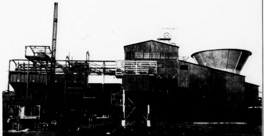
Fig. 2. Another construction photograph of the Coal Preparation Plant showing the large washing cone at the right. Heating a plant such as this requires a considerable amount of experience in estimating heat loss and in sizing and placing the heating equipment.
